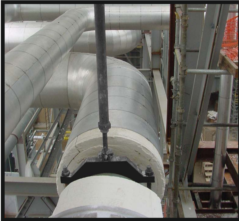
Rigid Strut with Fig RY3 stiff clamp
